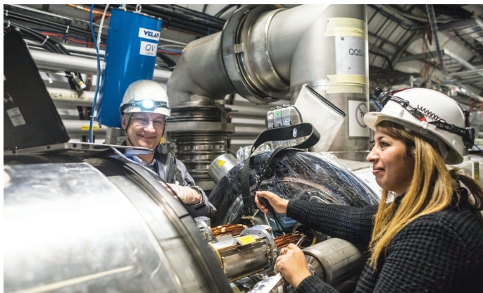
Electrical quality assurance on one of the 10 170 reinforced connections.
