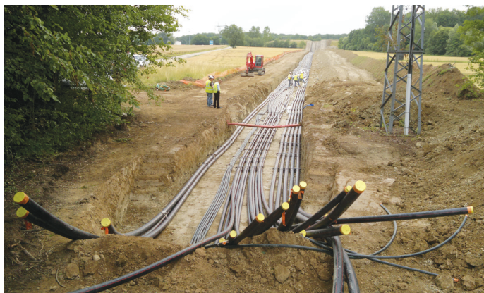
Replacement of the electrical distribution network for the SPS accelerator.
