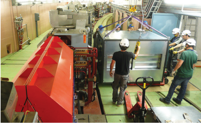
One of the new ventilation system stations for the PS is moved into the accelerator.
